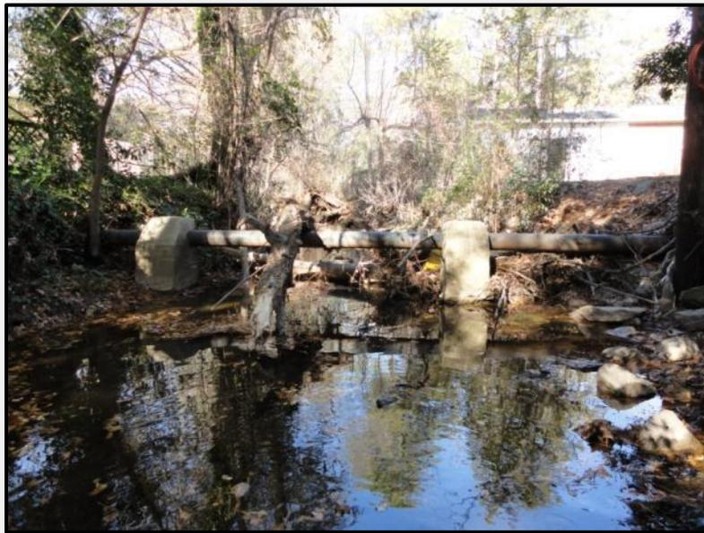
**Figure 15. Pipe crossing Kinley Creek with collected debris, immediately upstream of K-2 confluence. (USACE)**
