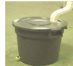
**Rain Barrels can capture and store runoff from the roof to be used later.**
